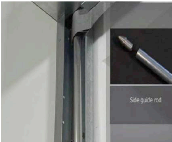
Curtain side pocket sliding over continuous rail to ensure fabric remains within side guide rail (shown during site assembly).
