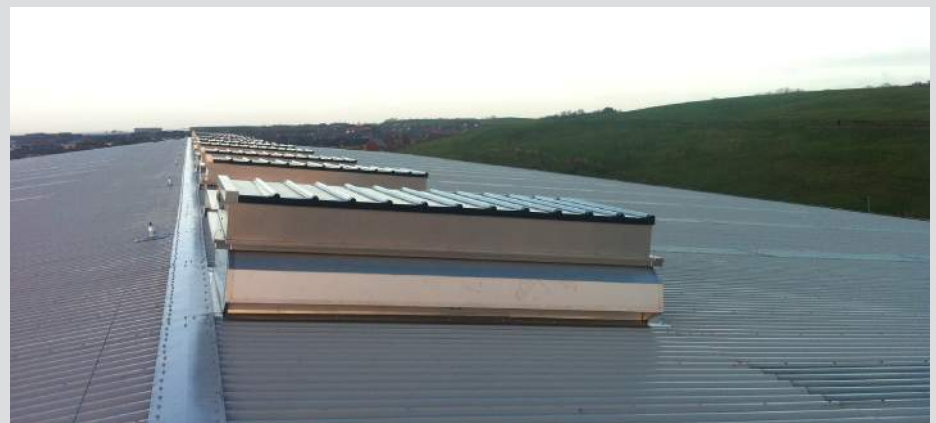
Weatherlite ventilated upstand at Chorley Parcelforce
